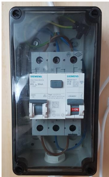
Modul 1e, Circuit Breaker and RCD
