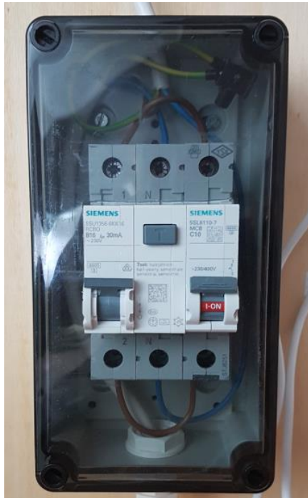
Module 1, Circuit Breaker and RCD
